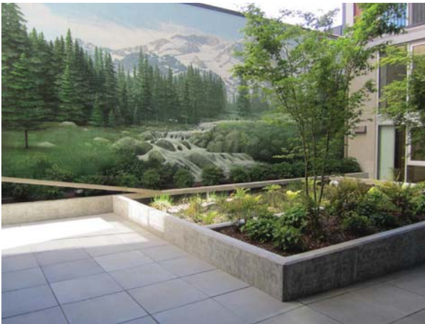
Stormwater Planter: H2O Apartments
